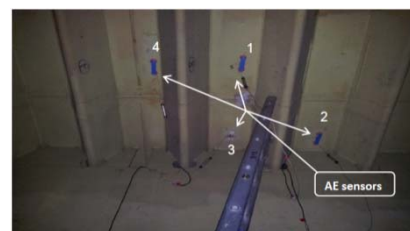
Figure 1: AE inspection site
