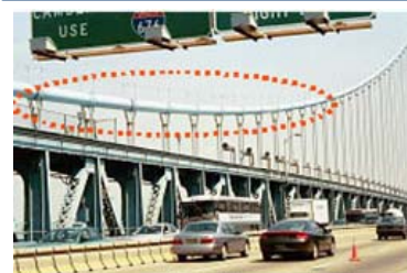
Figure 1. Acoustic Emission monitoring on a suspension bridge.
